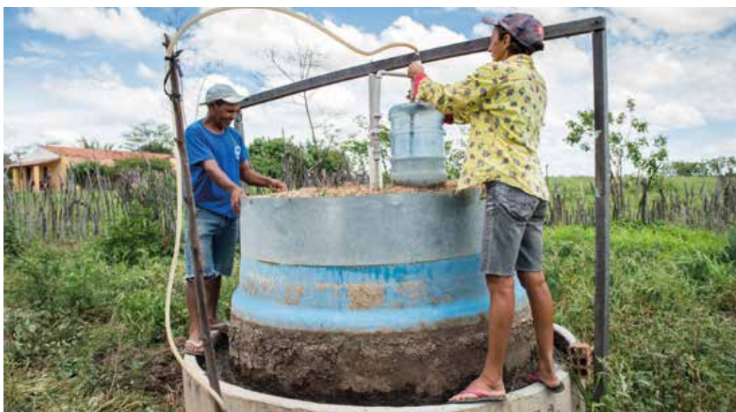
Biodigester turning waste into gas for cooking and fertiliser for farming in northeast Brazil. Eleanor Bentall/Tearfund
